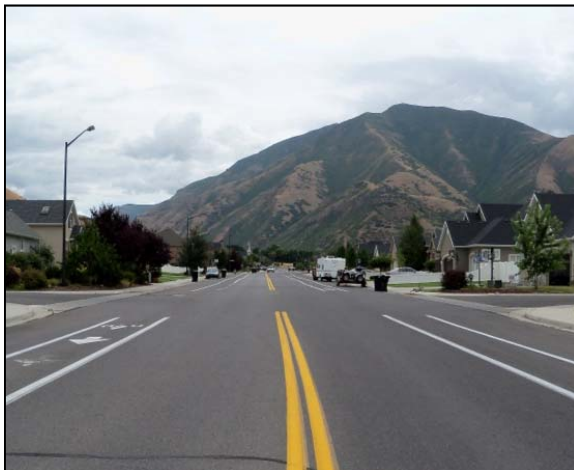
Figure 4-19 BEFORE: Illustration of River Bottom Road which is a wide residential Street
