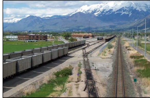
Figure 4-23 Three sets of rails run through Springville made, the City would be able to apply for the quiet zone with the FRA. Once a quiet zone is established, maintenance and continued compliance is required.
