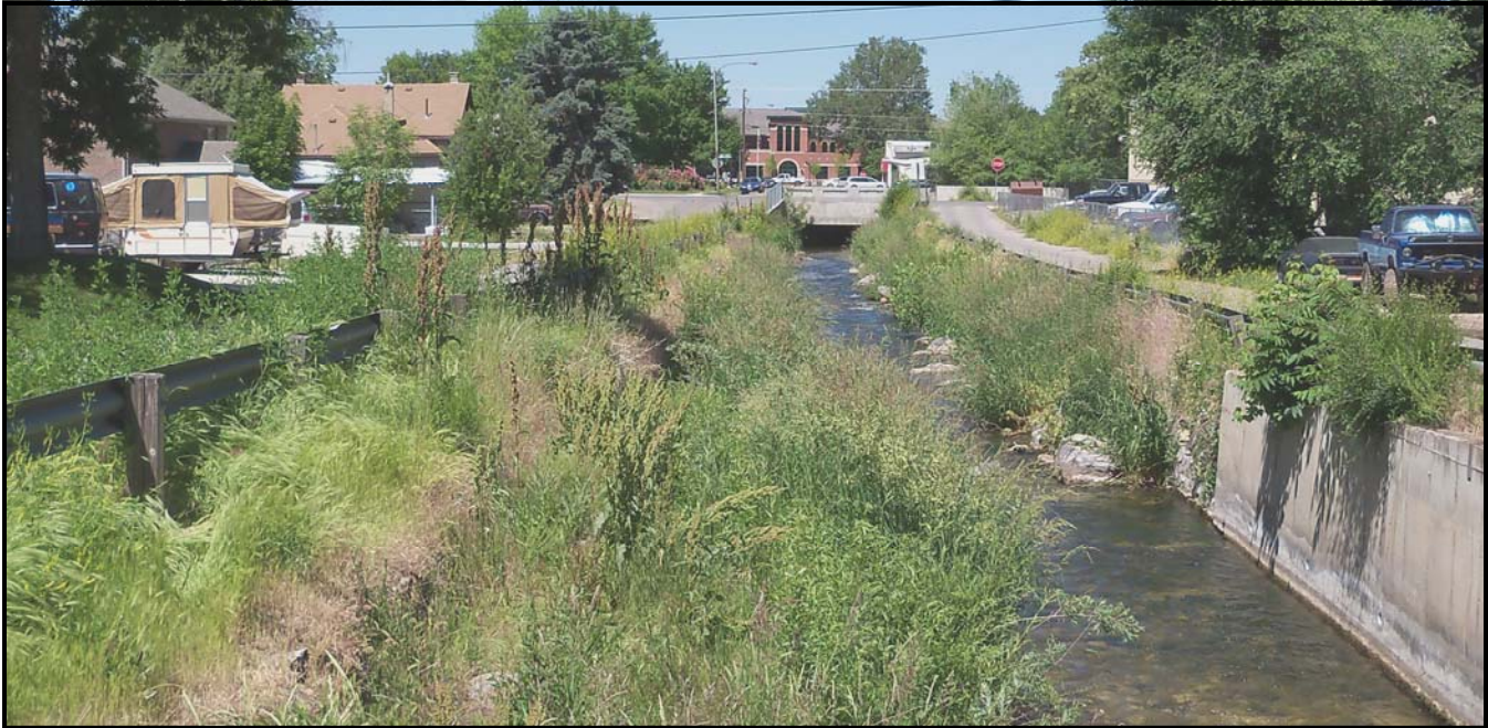
Figure 4-9 BEFORE: Hobble Creek running down 100 South between 100 East and 200 East
