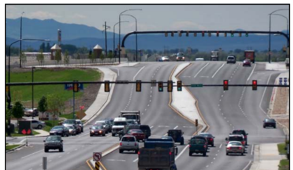
Figure 4-27 An example of an arterial located at the 400 South interchange
