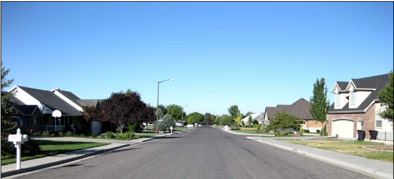
Figure 4-13 BEFORE: 700 South a long, wide, residential street with a 39' wide pavement surface.
