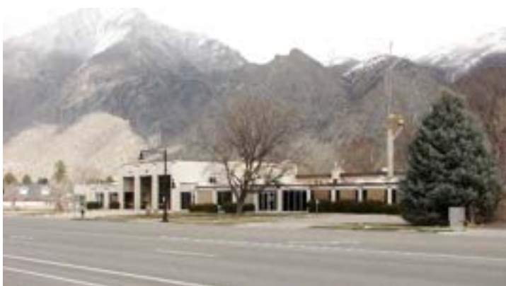
(The Fire Station and Police Station that was torn down. The Public Library is now on this lot)
