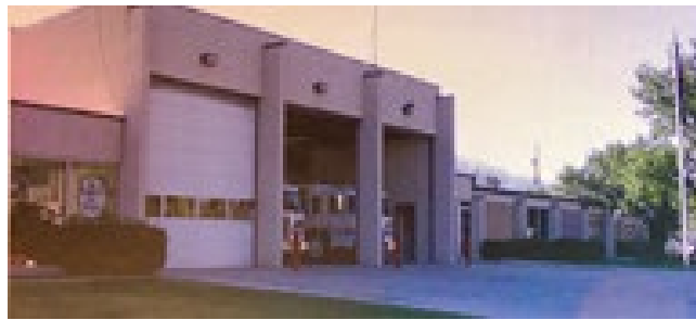
(Demolished Fire and Police Station, 45 S. Main St. Date unknown)
