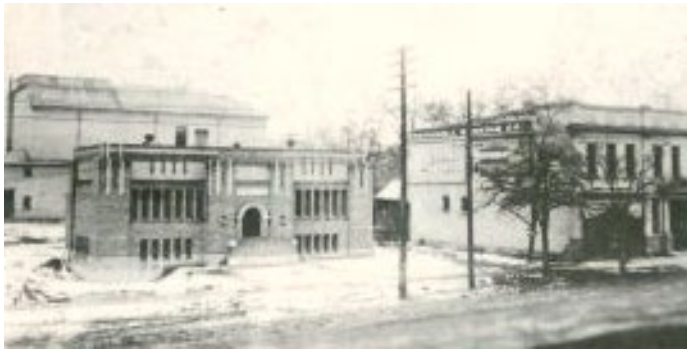
(Springville Carnegie Library. Date unknown)
