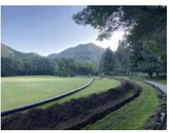
Over the summer the Hobble Creek Golf Course replaced the irrigation system on 114 acres of golf course property. The original irrigation system on the back nine was replaced, as well as the failing irrigation system on the front nine. A consolidation of the pump station and water source to the pump house and pond was completed between holes #1 and #7: and over 1.400
